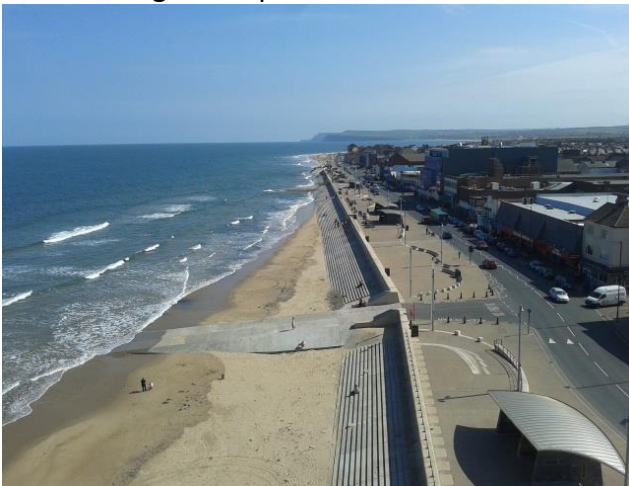
Figure 5. Sea walls at Redcar, NE England
