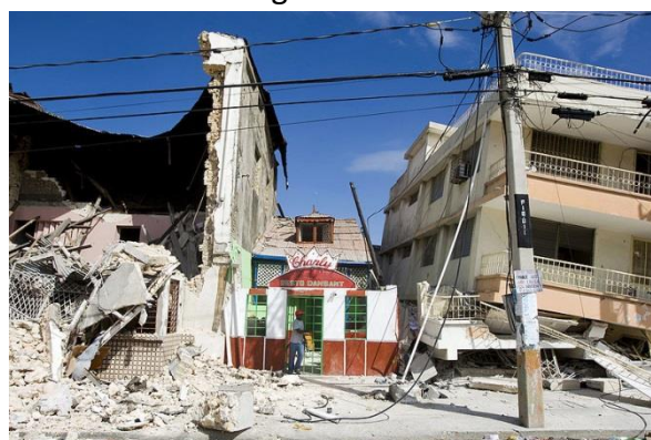
Figure 18 - building damage during the Haiti Earthquake By Photo Marco Dormino/ The United Nations United Nations Development Programme
