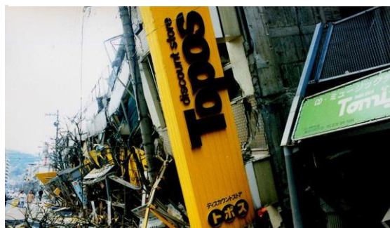
Figure 15 - damage during Kobe Earthquake By 松岡明芳 [GFDL ( http://www.gnu.org/copyleft/fdl.html )]
