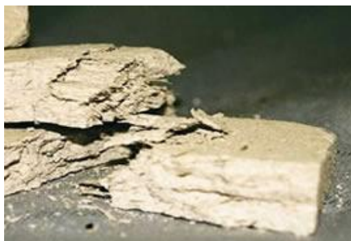
Pieces of Asbestos Insulating Board (AIB)
