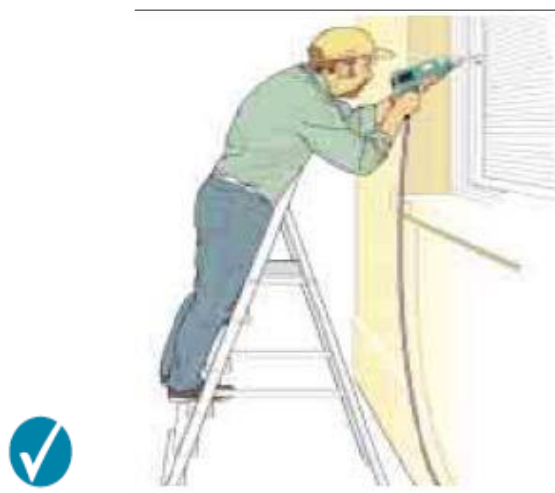
Correct – steps facing work activity
