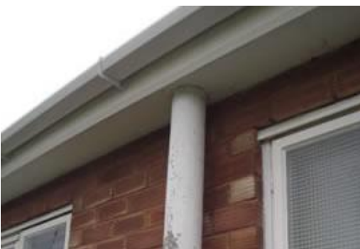
Asbestos cement drainage pipe (downpipe)
