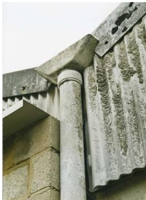
Asbestos cement downpipe, hopper and profile sheet
