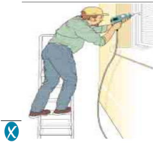
Incorrect – steps side on to work activity
