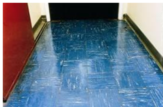
Asbestos containing floor tiles in a corridor
