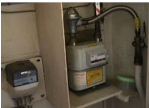
Asbestos panelling around a gas meter
