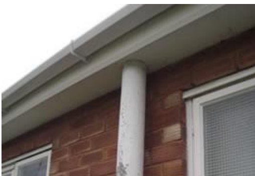
Asbestos cement drainage pipe (downpipe)
