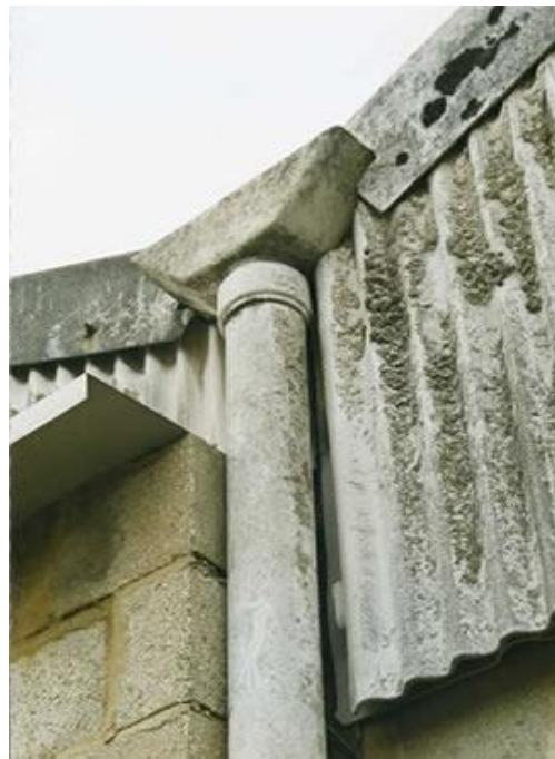
Asbestos cement downpipe, hopper and profile sheet
