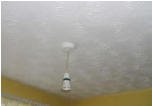
Asbestos textured coating
