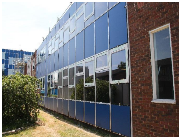
New windows and curtain walling installed (S1)
