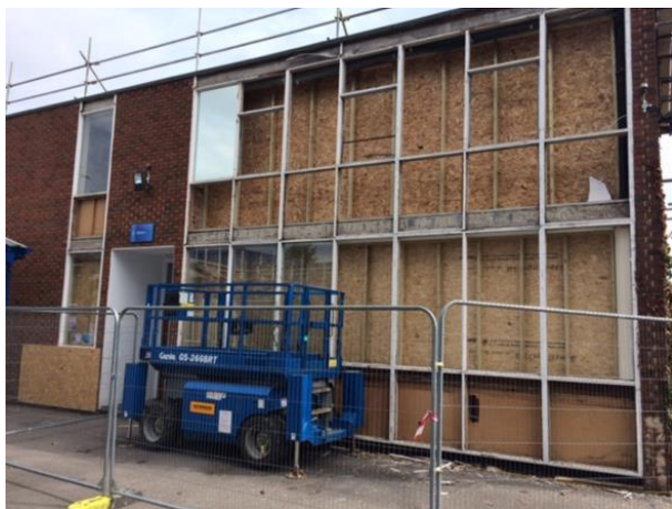
Old windows and curtain walling removed (S4)
