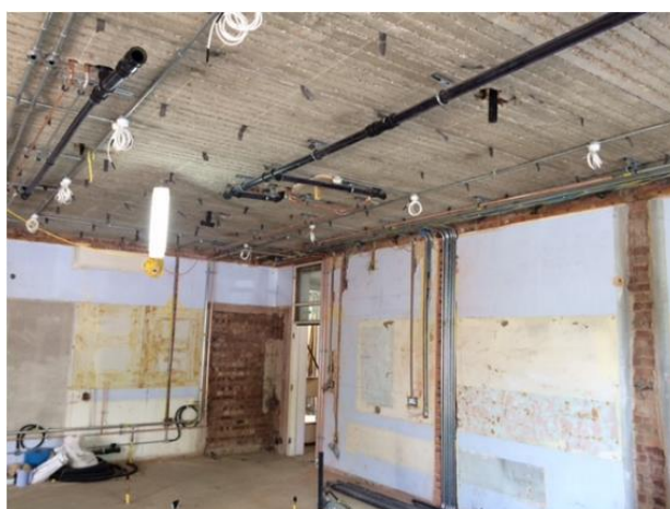
First fix of power, water and gas services
