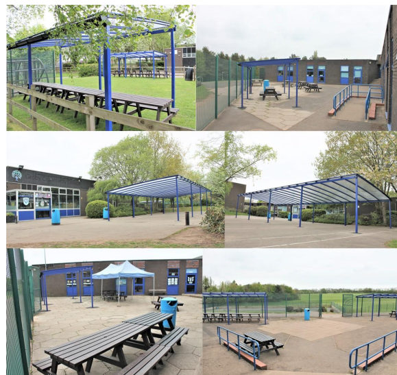
Installation of 7 new permanent sheltered areas & seating
