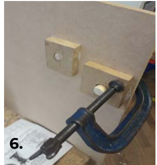
Here I have clamped the extra blocks to the main piece of MDF and have glued in the dowels with PVA. I checked with a try square to make sure they were all upright.
