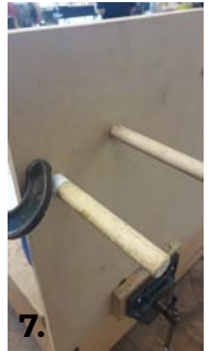
Here I have clamped the extra blocks to the main piece of MDF and have glued in the dowels with PVA. I checked with a try square to make sure they were all upright.
