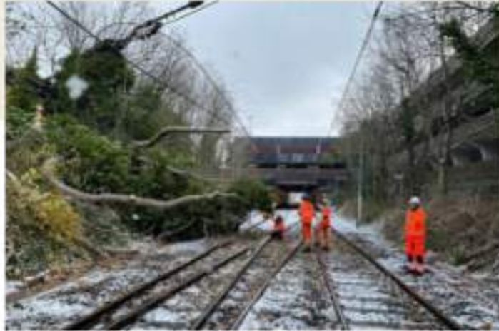
METRO MADNESS: The Metro had to be cancelled all day on Saturday and Sunday because Storm Arwen had caused trees to fall over and block the train track.
