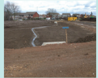
An example of a large basin under construction.
