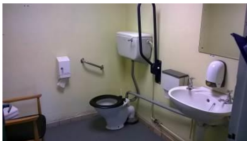
P014 – Accessible toilet not compliant.
